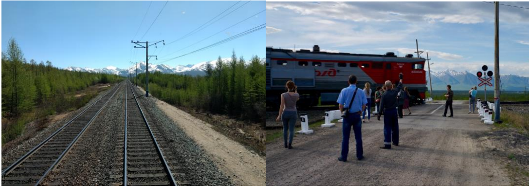
Picture 1: Railway tracks on the way to Mururin Pass, the highest point of the terrain traversed by the BAM (Stefan Sametinger)
